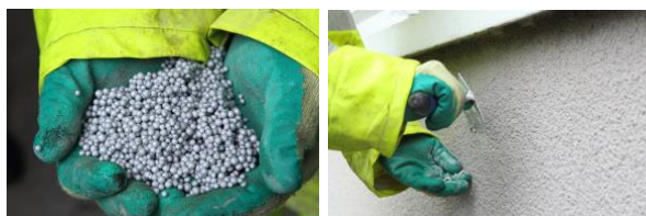
Cavity wall 'beads' and post installation finishing
