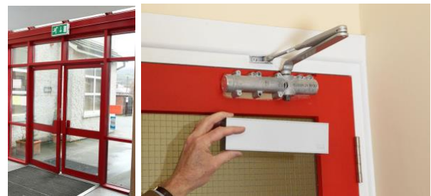
Ensure doors close properly. Fit adjustable door closers
