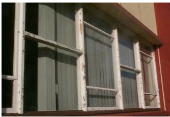
Single glazed timber window
