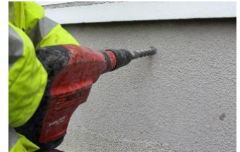
Cavity wall installation
