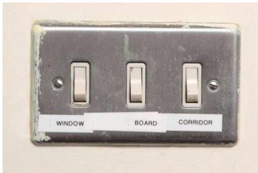
Label light switches
