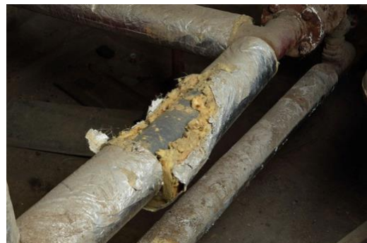
Repair damaged insulation
